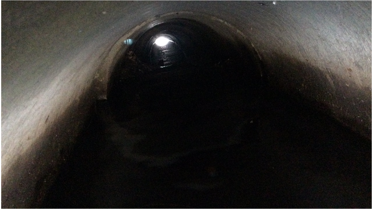
View of culvert on the inside.
